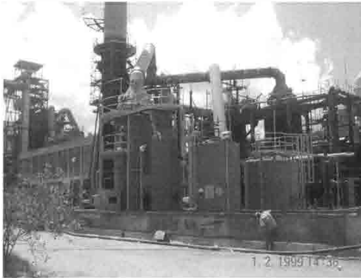
Peracidox Plant - Brazil
