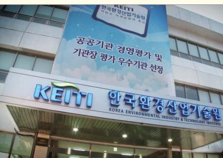
● Office building of KEITI
