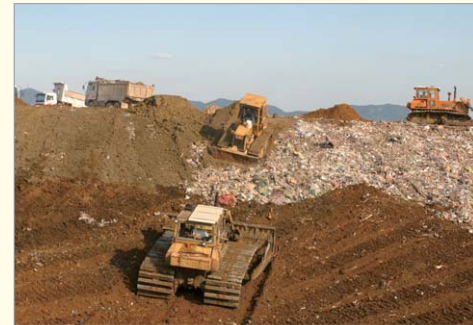
● Soil Covering Process during Sanitary Landfill
