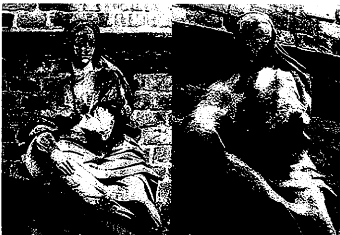
How acid rain affects stonework. The picture on the left was taken in 1908. The picture on the right was taken in 1968
