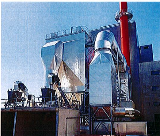
2-Field ESP with ERCS plant
