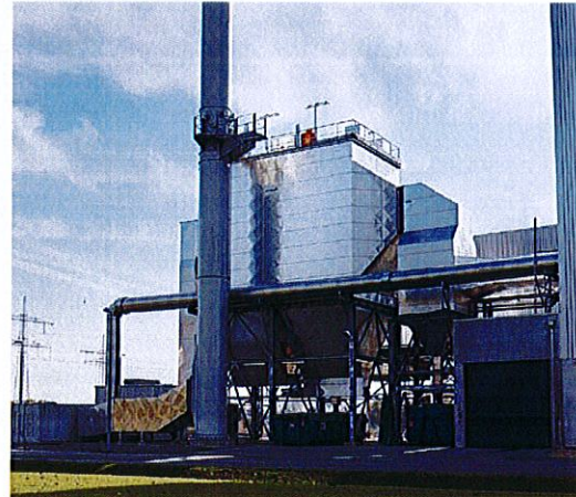
2-Field ESP with multi-cyclone
