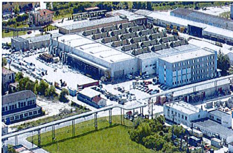
Branch Office with Workshop - SCHEUCH s.r.o. Prievidza/Slovakia
