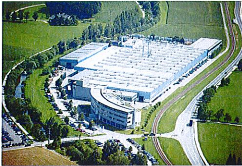
Company Headquarters - SCHEUCH GmbH Auroszmünster/Austria
