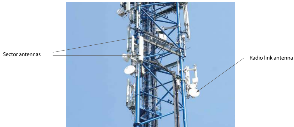
Fig. 4. Types of antennas in a mobile telephony base station. Source: own NIT data
