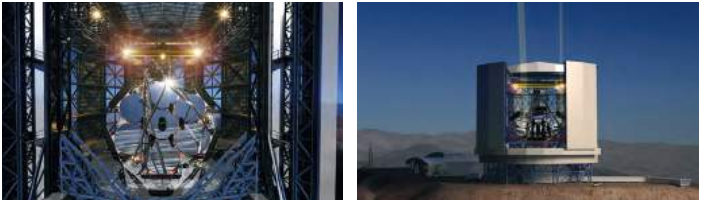
Figure 5. Two artist conceptions of the GMT telescope, showing the seven mirrors in a single structure and the enclosure. Notice several objects placed in the images for scale comparison. The laser beams emerging from the telescope in the right-hand picture are part of a complex system called Adaptive Optics (AO), used to compensate for the effects of the atmosphere's turbulence. © Giant Magellan Telescope – GMTO Corporation.
