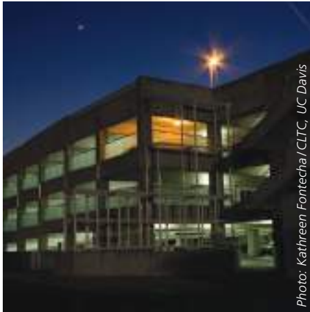
Figure 10. Adaptive parking garage lighting at UC Davis employs both occupancy and daylighting controls. In California, there are now requirements for both to be included in most lighting alterations for parking garages.
