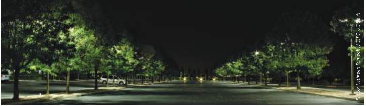
Figure 14. UC Davis parking lot with adaptive induction lighting
