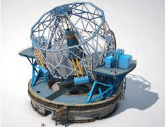
Figure 7. Artist conception of the E-ELT. The blue boxes, to the right of the telescope correspond to just one of the instruments. Also shown is an example of 5 out of almost 800 segments. © ESO, licensed under CC BY 4.0.
